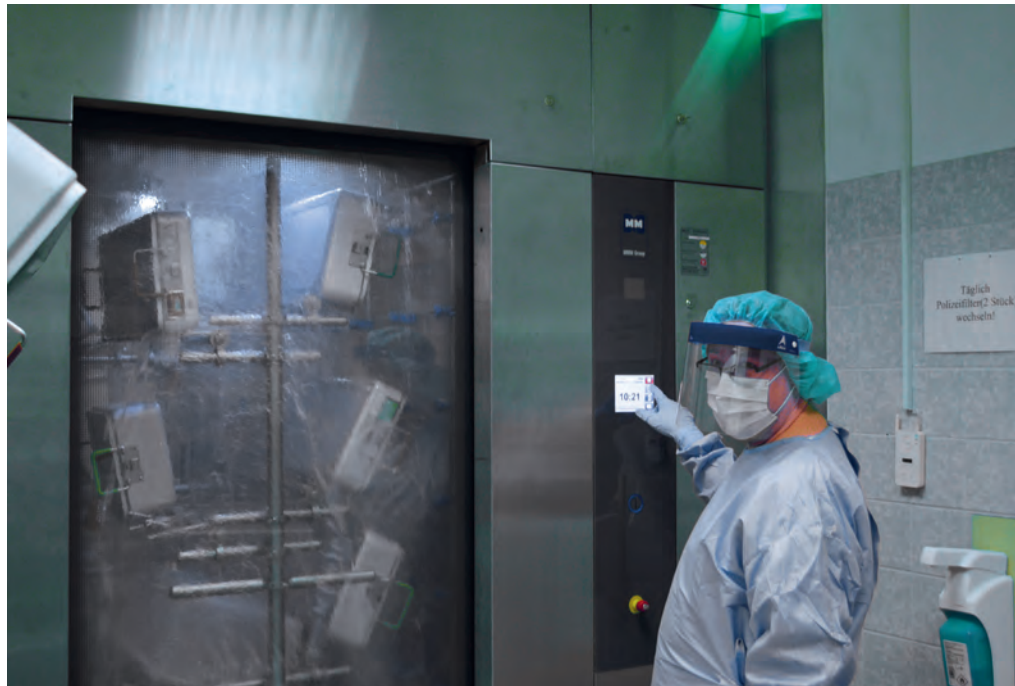
Fig. 2: Commissioning of the container washing facility, using the cleaner neodisher® MediClean forte and the rinsing agent neodisher® MediKlar. Within the validation process, protein soiling of 0 µg were detected in 6 of 8 cleaning runs.
